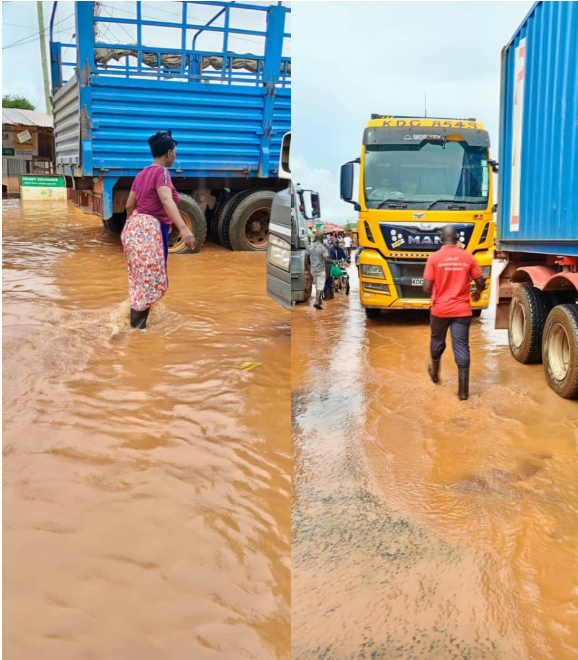
A section of the main road towards the One Stop Border Post.
